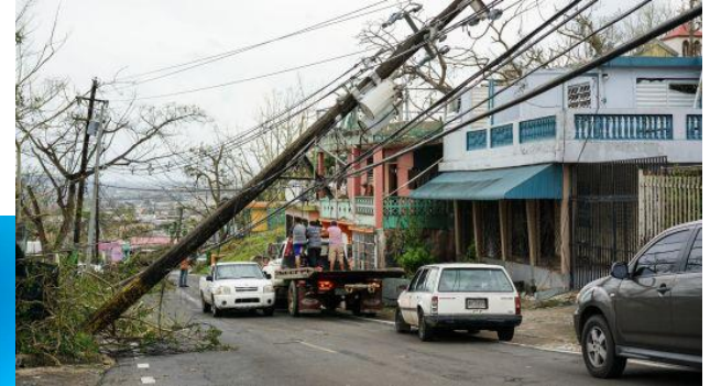
Hurricane Maria, Puerto Rico 2017
