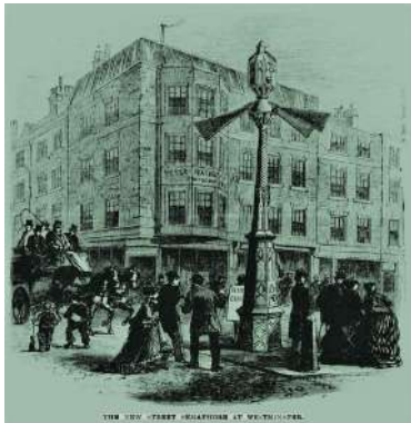
Figure: First signal control in the world, January 16, 1869 installed in Westminster, London
